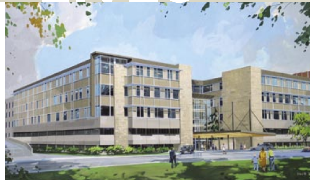
The redevelopment of Kingston General Hospital includes the addition of three floors to the Burr wing for cancer, renal and acute mental health care.
